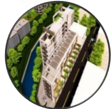
Promotion of BCR Construction Projects
