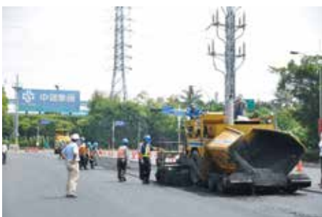
Road paving with BOFS asphalt concrete
