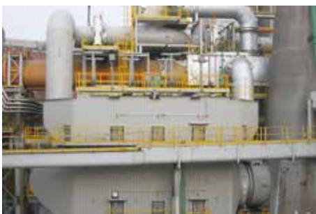
The waste heat recovery equipment at the No. 1 Blast Furnace
