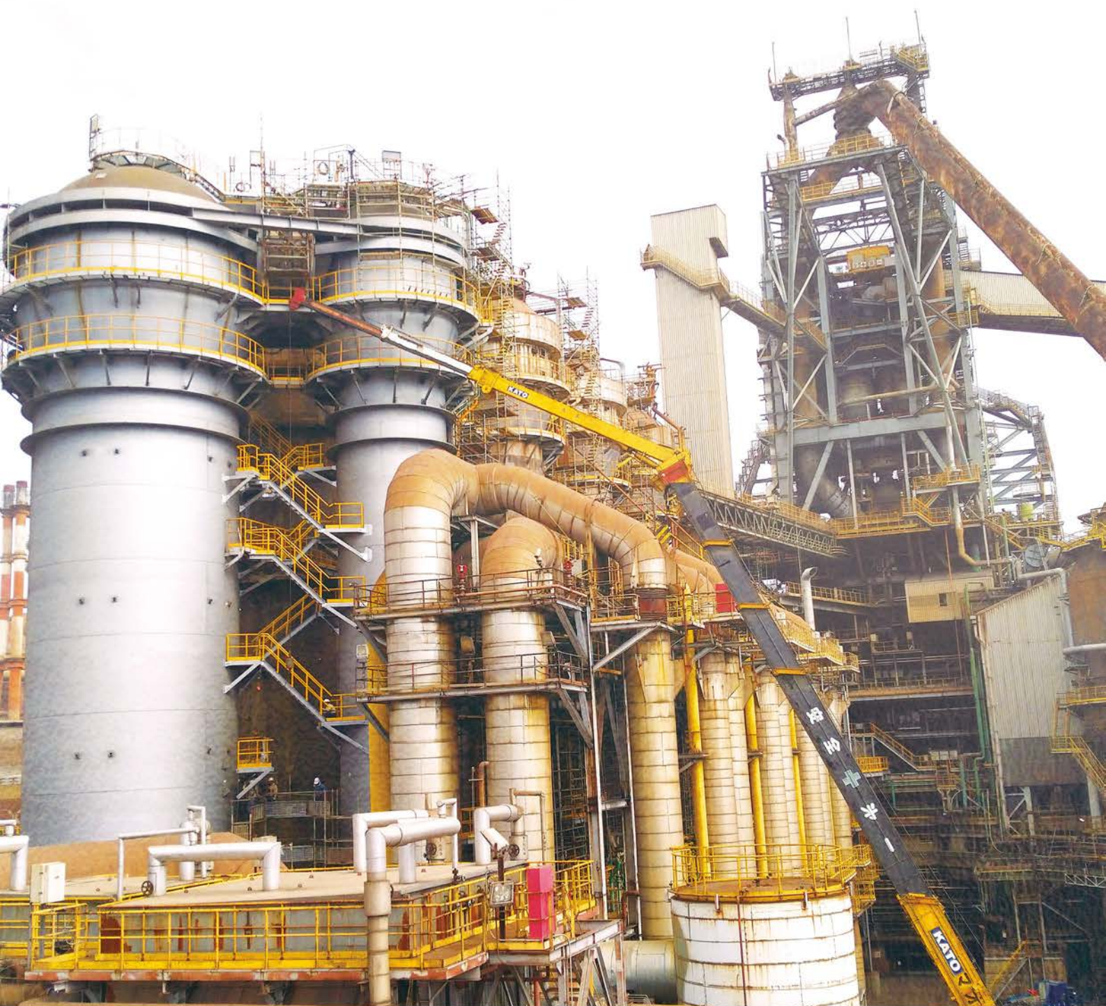
No. 34 hot stove in the No. 3 Blast Furnace
