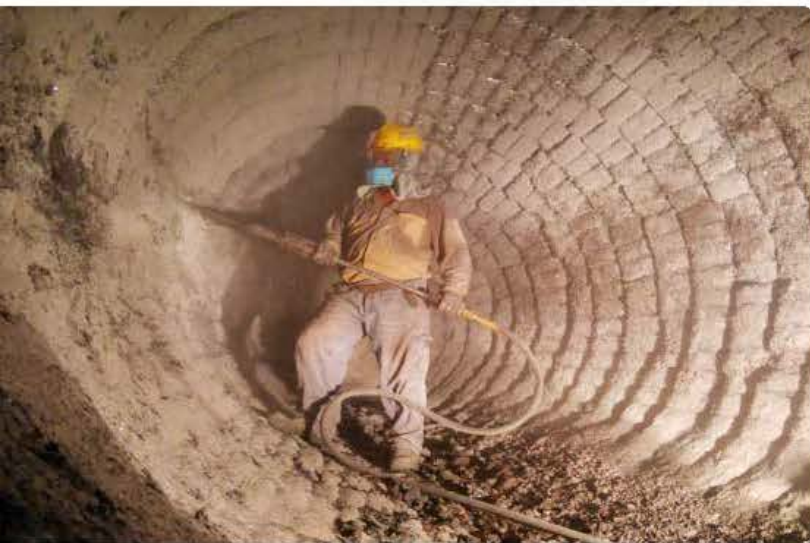
Deslagging inside a torpedero car
