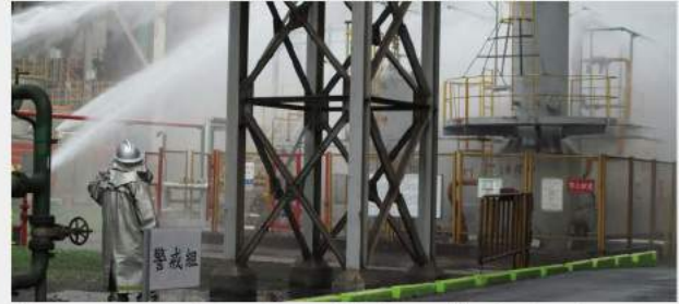
When an ammonia leakage in a tank is detected by the detection system, water is sprayed immediately to prevent the massive diffusion of ammonia.
