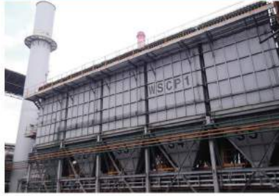
No.1 waste scrap cutting plant dust collector
