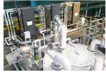
The waste water recycling system in the electrogalvanizing lines
