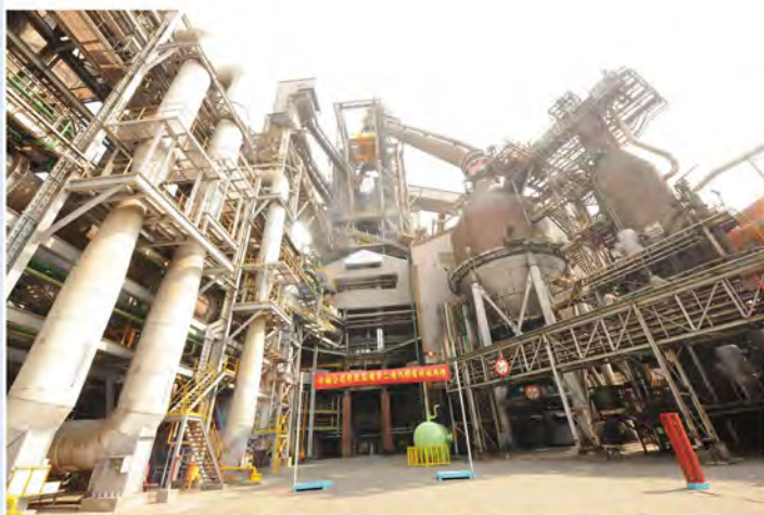
The blow-in of the second campaign of CSC's No.4 blast furnace
