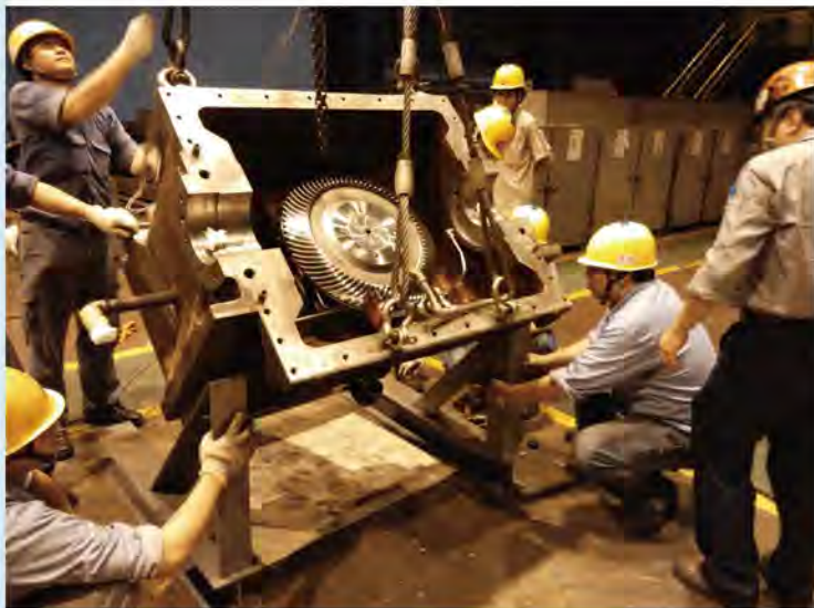
Repairs of equipment
