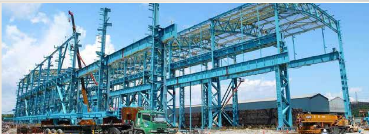
Construction in progress of the non-oriented electrical steel production line
