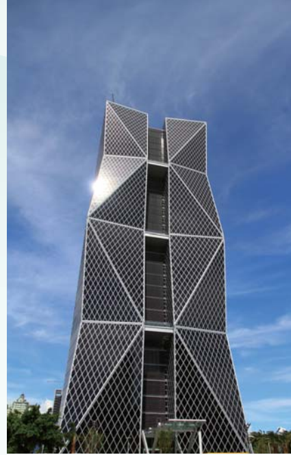
China Steel Building was constructed by building structure steel SN490B and SN490C.
