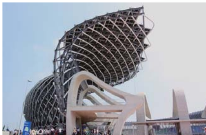
National Stadium of Kaoshiung is constructed by CSC's building structure steel SN490A and high strength structural steel A572 Gr.50.
