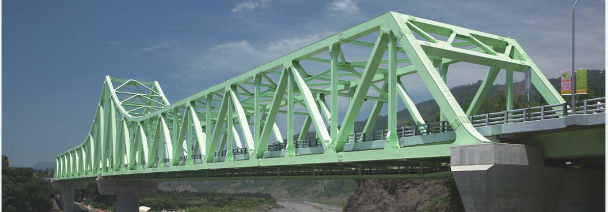
Xinfa bridge, which was donated and constructed by CSC Group, was built by atmospheric corrosion structural steel for bridge A709 Gr.50W.
