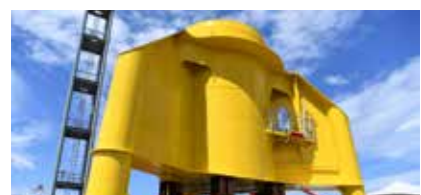
Taiwan's first transition piece mock-up to a jacket foundation
