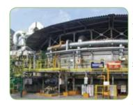
CSC launched the rotary hearth furnace (RHF) process in 2008. It increased the recycling volume of dust and sludge while decreasing the emission of dioxin in sinter plants by converting them into high value-added Direct Reduction Iron (DRI) for BF and ZnO powder(Zn>50%), which are sold to zinc refineries in Japan.
