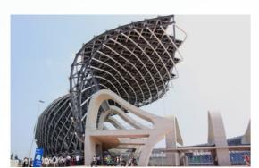
National Stadium of Kaoshiung is constructed by CSC's building structure steel SN490A and high strength structural steel A572 Gr.50.
