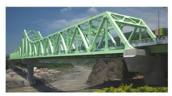
Xinfa bridge, which was donated and constructed by CSC Group, was built by atmospheric corrosion structural steel A709 Gr.50W.
