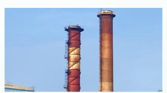
One of CSC plant site chimneys was made from corrosion resistant steel SCR-TEN.
