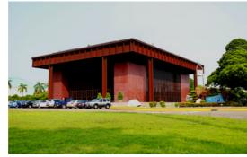
China Steel auditorium was constructed by atmospheric corrosion resistant structural steel A588.
