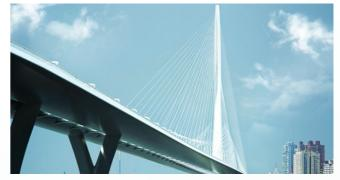
Danjiang Bridge located in Tamsui, Taipei was built by high performance atmospheric corrosion resistance structural steel A709 Gr.HPS 70W.
