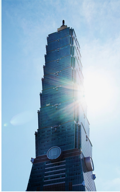
Taipei 101 Building was constructed by using steel SM570M for welded structures.
