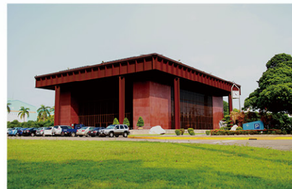
CSC auditorium was constructed by atmospheric corrosion resistant structural steel A588.
