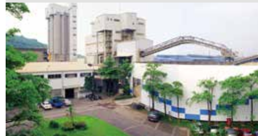
爐石粉研磨廠 (高雄總廠)
