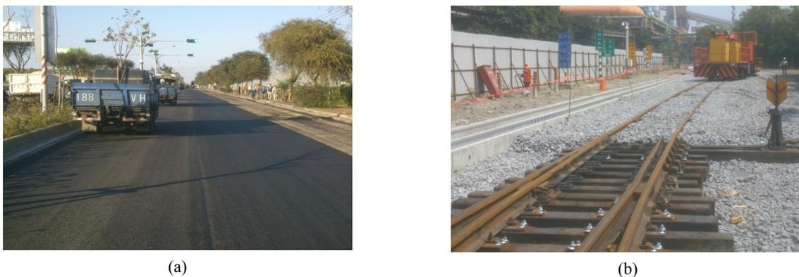
**Fig.8.** (a) The road with the length of 1.2 km was paved by modified BOF slag-based AC in Tainan city of Taiwan, (b) Modified BOF slag was utilized in the railway ballast of torpedo car at CSC.
