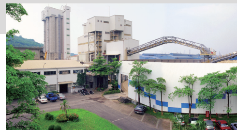
爐石粉研磨廠 (高雄總廠)
